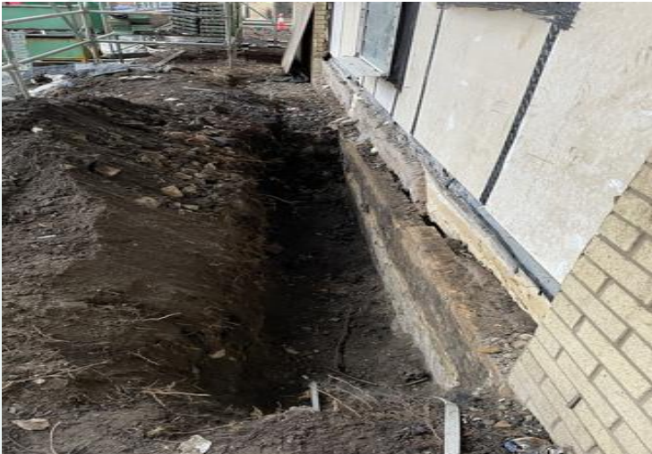
Blockwork foundation
